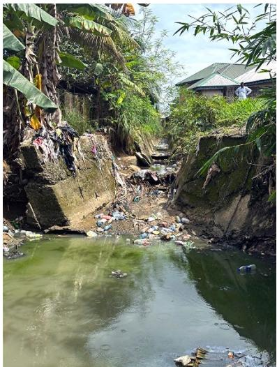
A serious erosion problem is threatening the buildings on the Calabar church/school compound and their neighbors due to a broken gutter. Water from an adjoining neighborhood is passing through the compound. A wall and part of the baptistry have been lost due to this erosion. Several appeals have been made to the responsible departments of the city government but no response has been received.
